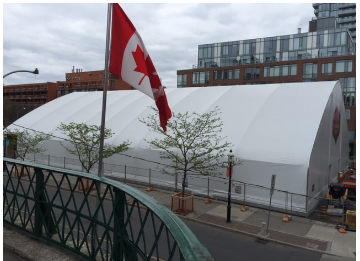
Figure 4. Building structure completed including insulated fabric cover.
