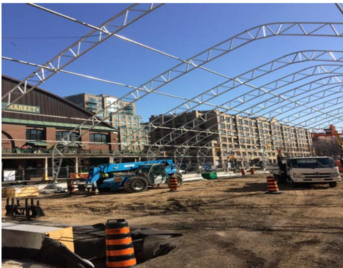
Figure 3. Site work completed and backfilled. Steel truss framing installation underway.
