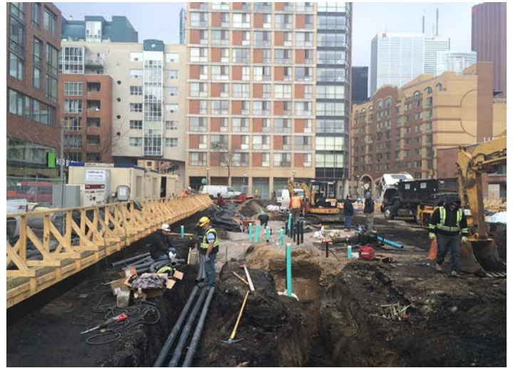
Figure 2. Site servicing work.
