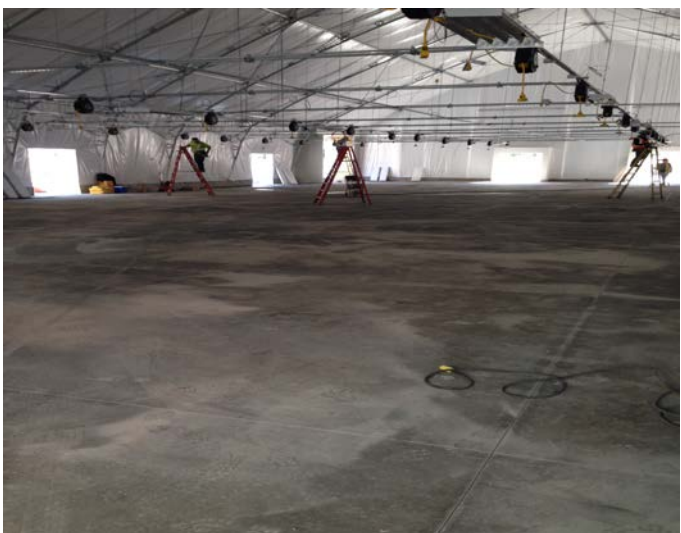
Figure 5. Interior fit-out nearing completion.
