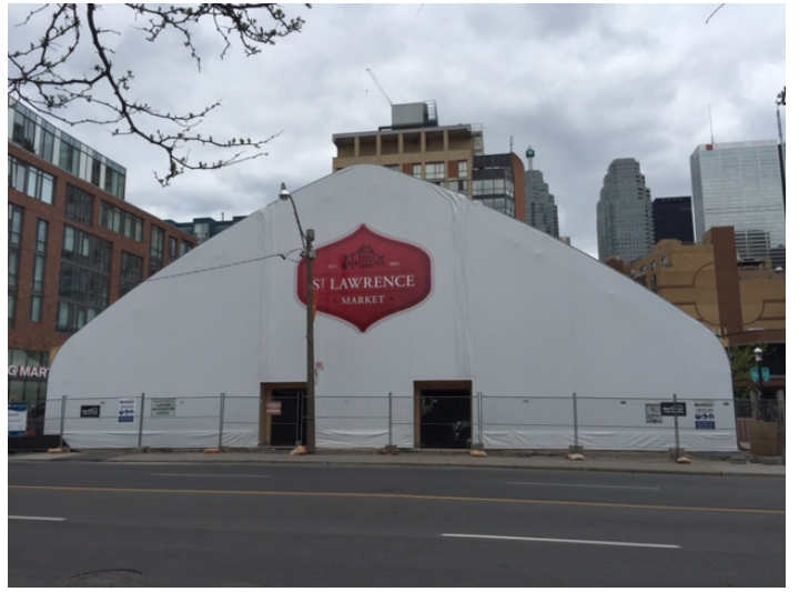
Figure 6. Exterior construction nearing completion.
