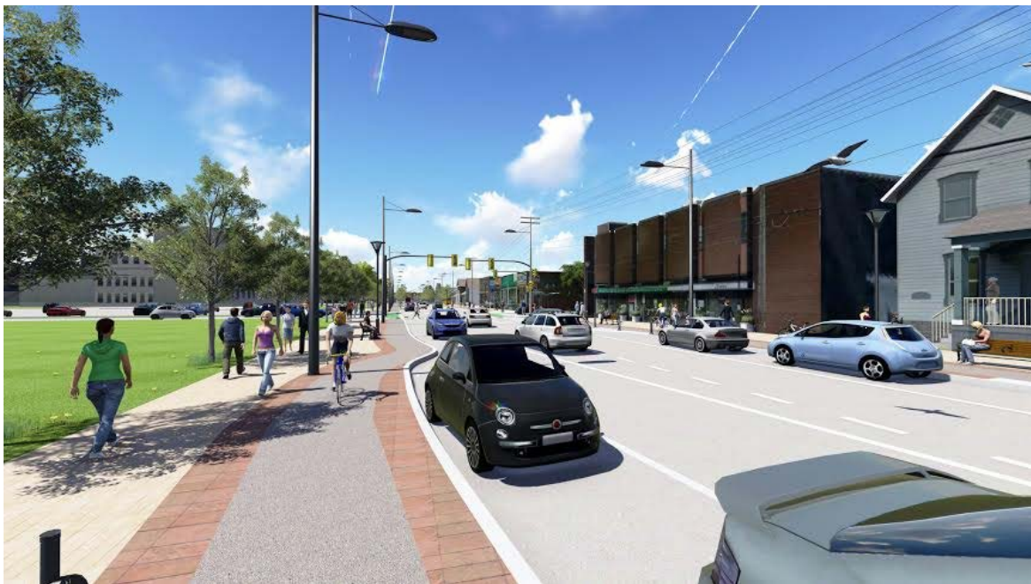
Figure 5: Ottawa cycle track at sidewalk level – Main Street (Photo Credit: Kornel Mucsi, City of Ottawa)
