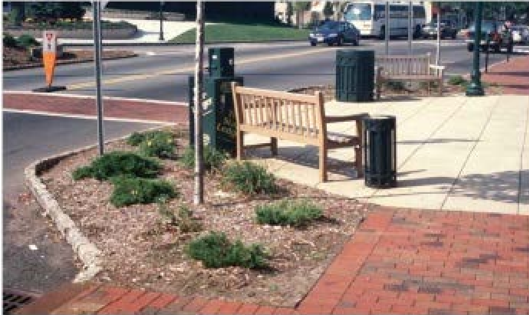
Figure 6: San Francisco curb extensions (Photo Credit: “Better Streets” website: “Intersection Design: Design Features: Curb Extensions (Bulb-outs)”, City and County of San Francisco: http://www.sfbetterstreets.org/design-guidelines/intersection-design/ )
