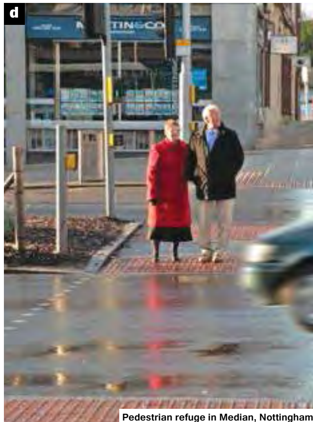
Pedestrian refuge in Median, Nottingham
