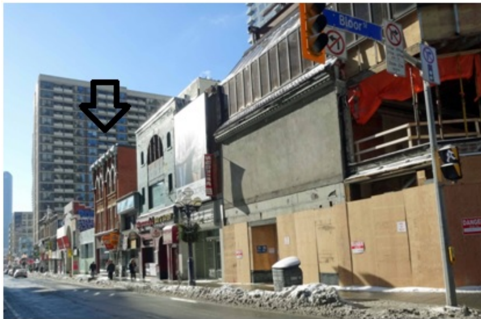
16. Current Photographs, 774 Yonge Street, 2015 : showing the east elevations and north side wall of the William Luke Buildings (above) and their context on the west side of Bloor Street, south of Yonge Street ((below) (Heritage Preservation Services)
