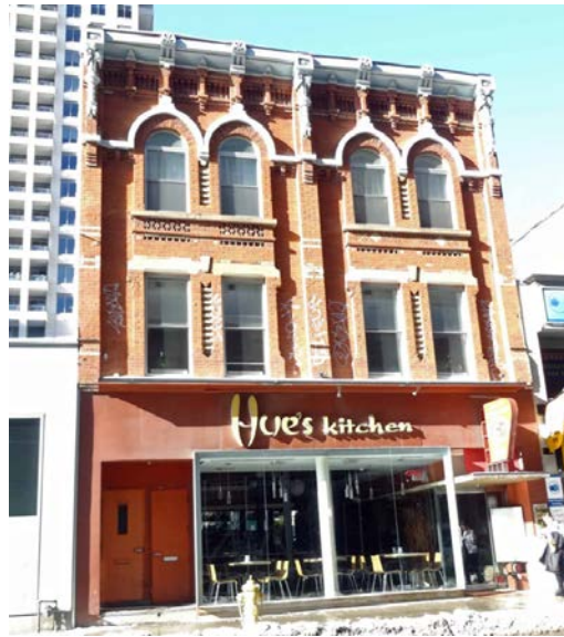
Above: west elevations of the William Luke Buildings; cover: view of the properties at 774 Yonge Street on the west side of the street, south of Bloor Street West (Heritage Preservation Services, 2015)
