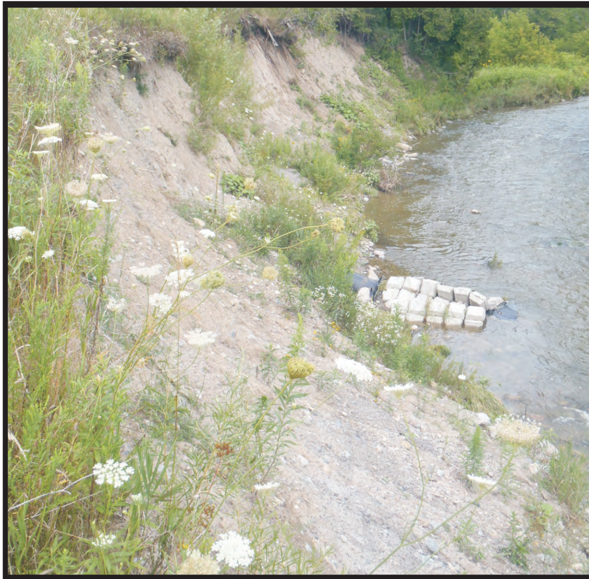
Photo of interim stabilization measures at exposure of Line 9B pipeline at the Rouge River.
