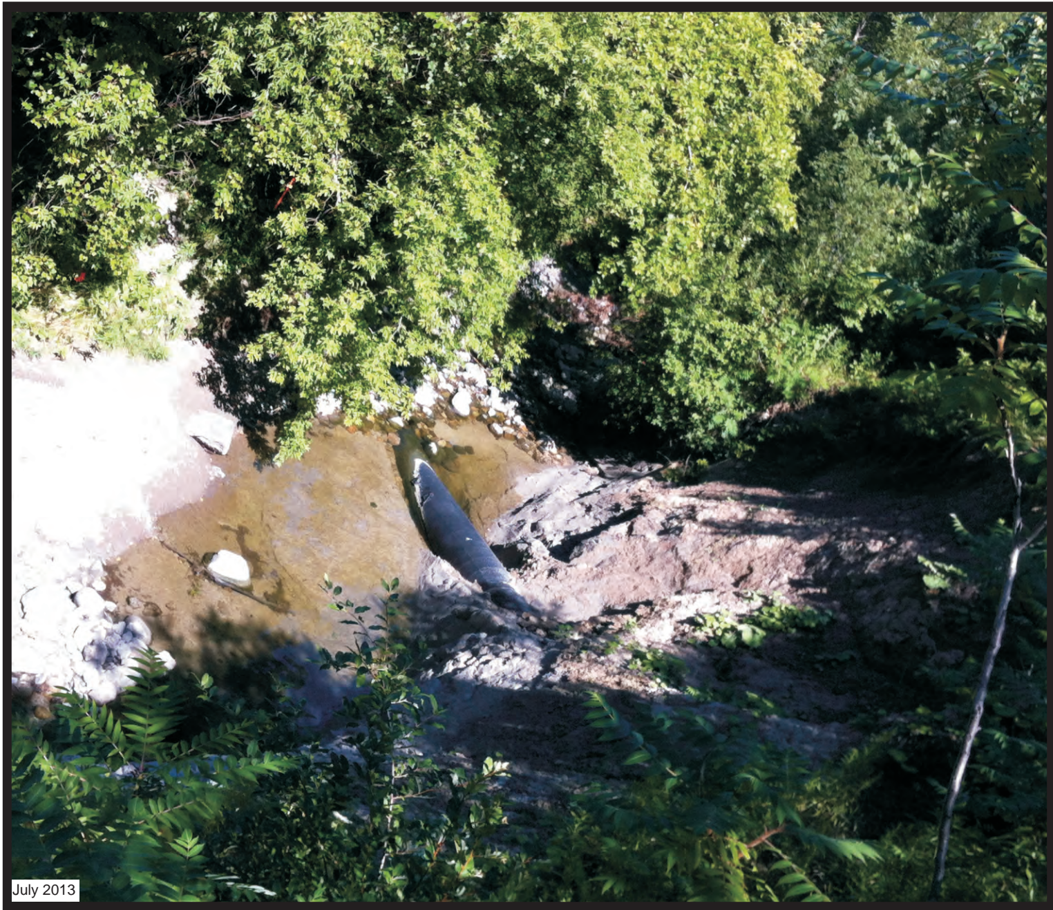
Photo of exposed Line 9B pipeline within Newtonbrook Creek - Don River Watershed
