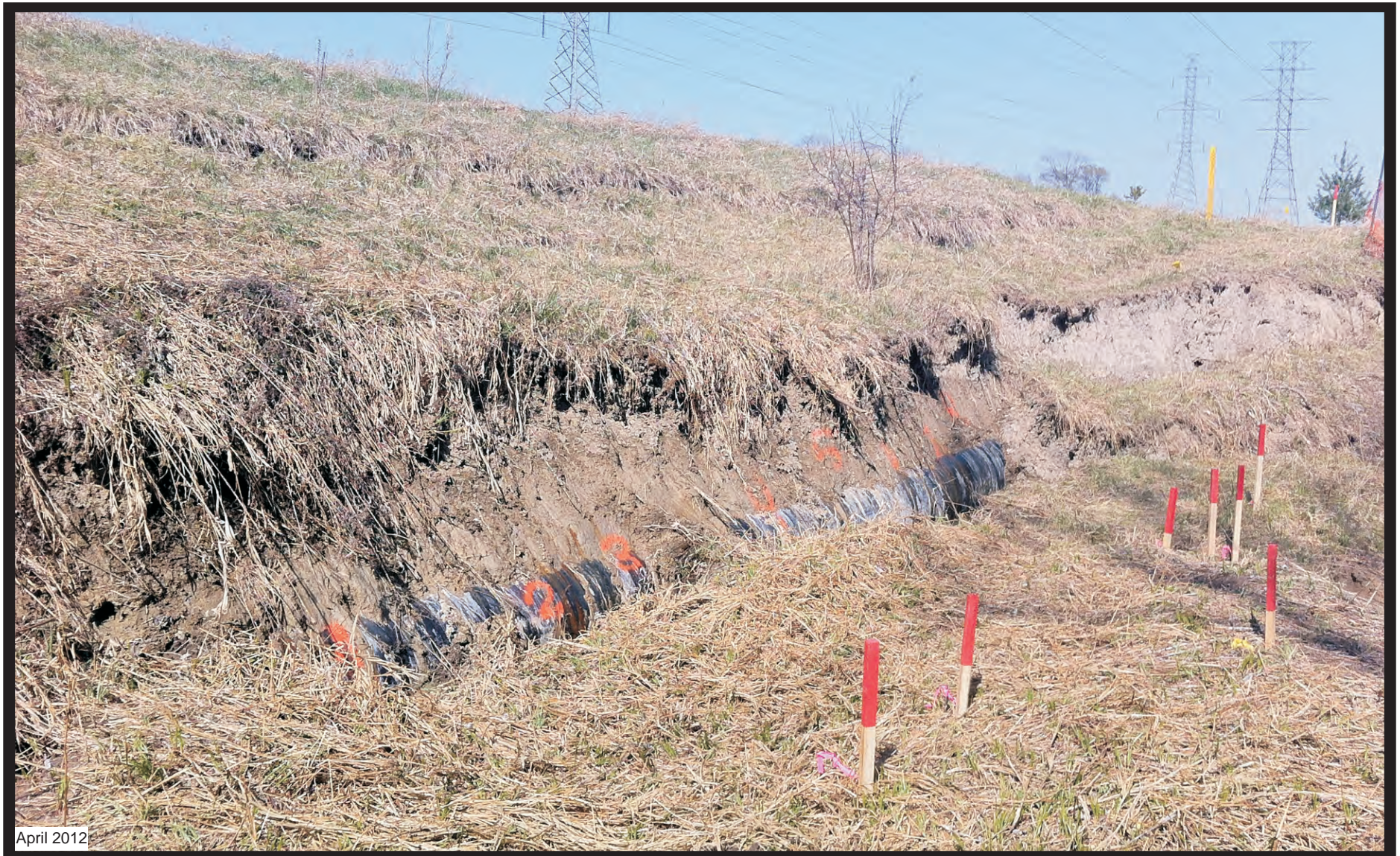
Photo of exposed Line 9B pipeline adjacent to the East Don Provincially Significant Wetland (PSW) Complex
