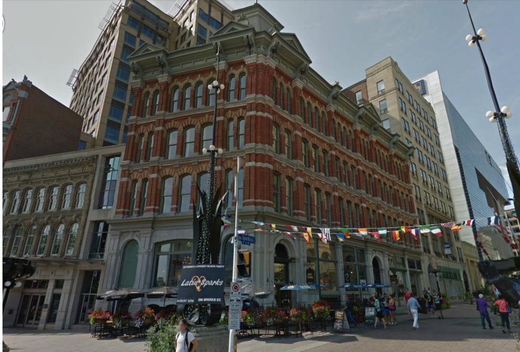
9. Scottish Ontario Chambers, 42-50 Sparks Street, Ottawa : also constructed by the Scottish Ontario and Manitoba Land Company in 1883, architect William Hodgson. ( Google, August 2014 )
