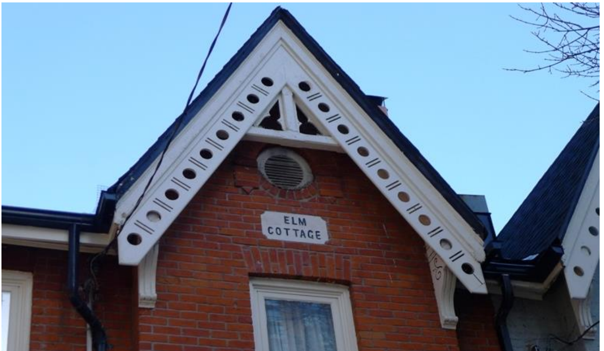
14. Elm Cottage, gable roof bargeboard detail . ( Heritage Preservation Services 2015 )
