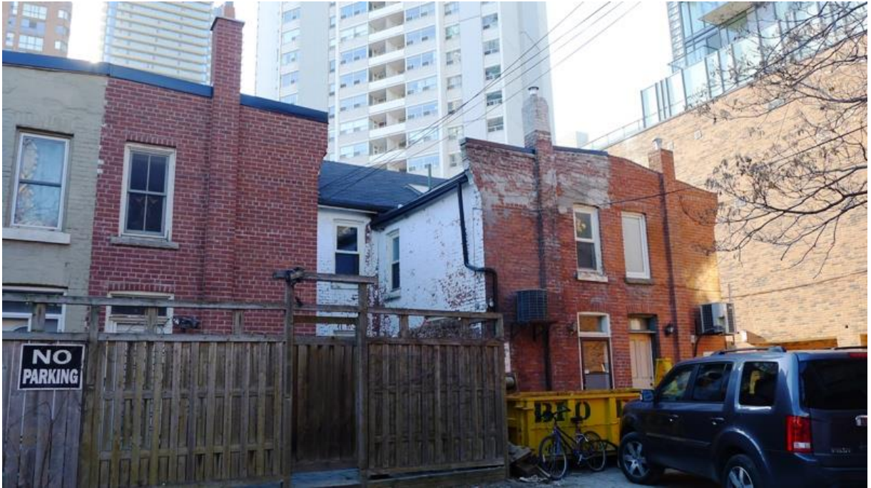
13. 57-63 St. Nicholas Street : showing the rear two story additions and the L-shaped massing of the houses. ( Heritage Preservation Services, 2015 )
