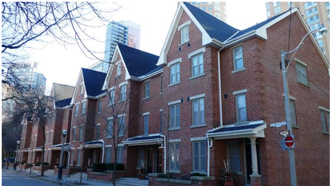
22. 50-84 St. Nicholas Street : showing the new condominium development with its four storey height and elements from the 1883 row houses including the gables, bays and sloping roof porches and small setback for landscaping and trees. (Heritage Preservation Services, 2015)
