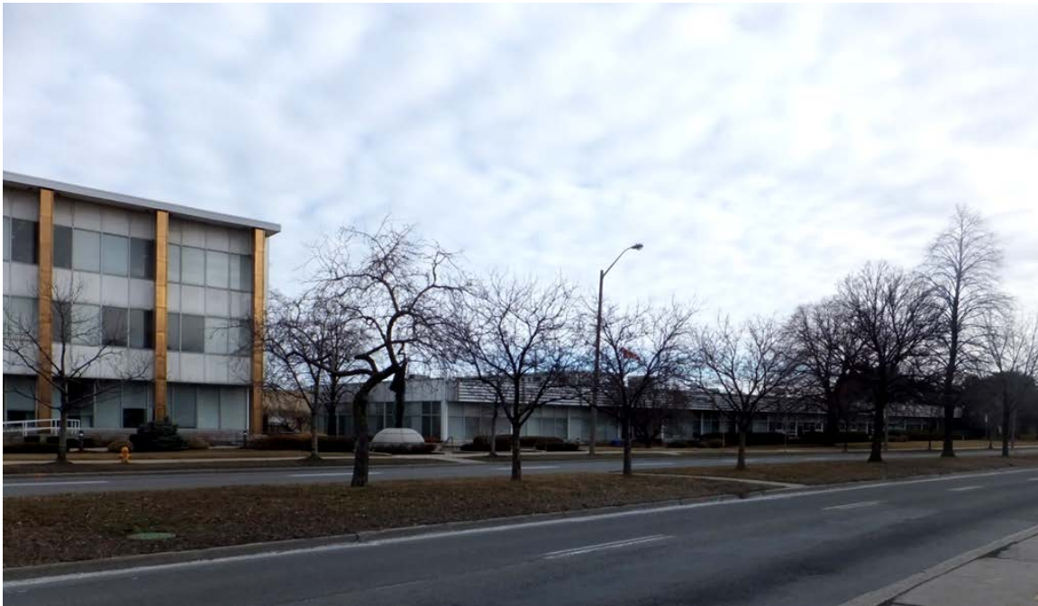
16. Photographs : looking west (above) and east (below) on Overlea Boulevard and showing the Coca-Cola Building in relation to the adjoining bottling plant (right) that was demolished in 2014 (Heritage Preservation Services)
