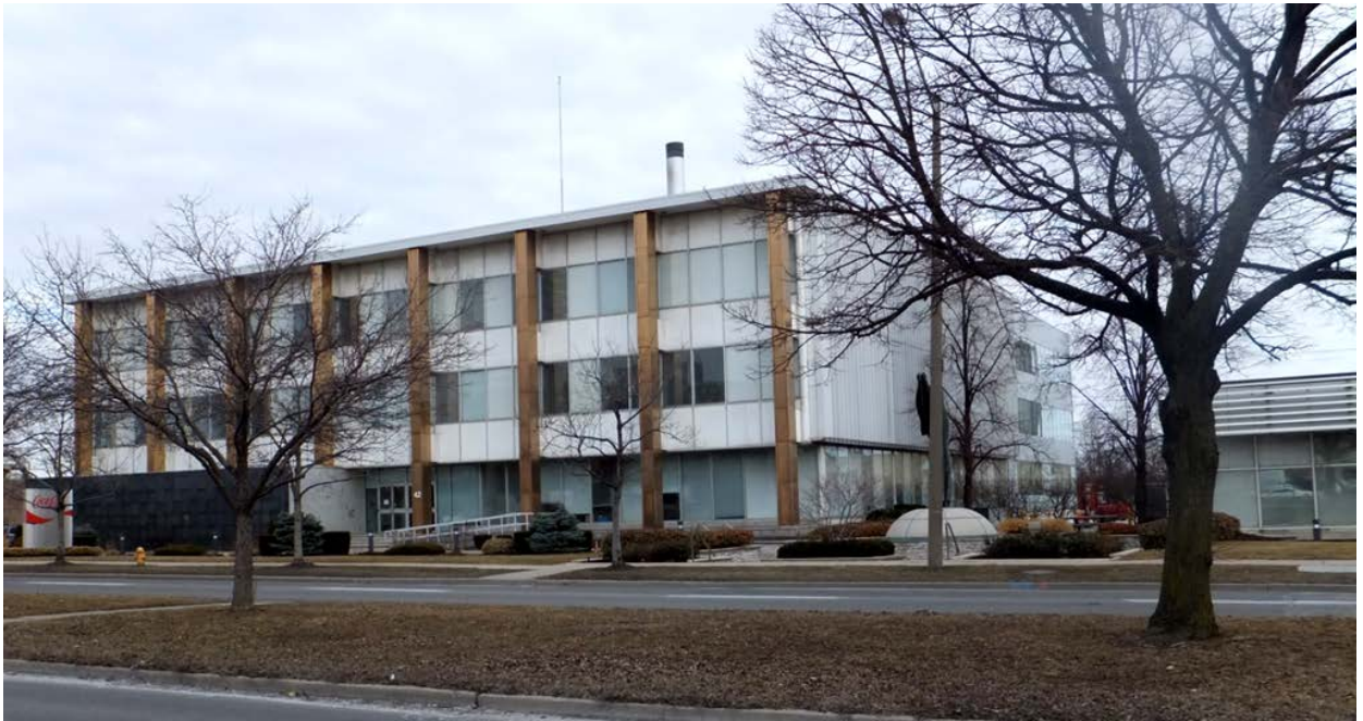
13. Photographs: showing the west (left) and south (right) elevations (above) with the south (left) and east (right) elevations (below) prior to the demolition of the bottling plant (right) (Heritage Preservation Services)
