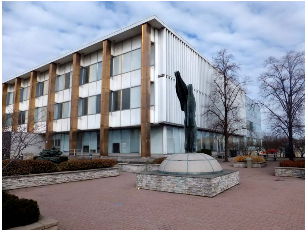
15. Photographs : showing the setback of Coca-Cola Building on north side of Overlea Boulevard before the demolition of the neighbouring bottling plant (above), and the adjoining courtyard with the "Coca-Cola" sculpture by Walter Yarwood that was removed from the property in July 2015 (Heritage Preservation Services)
