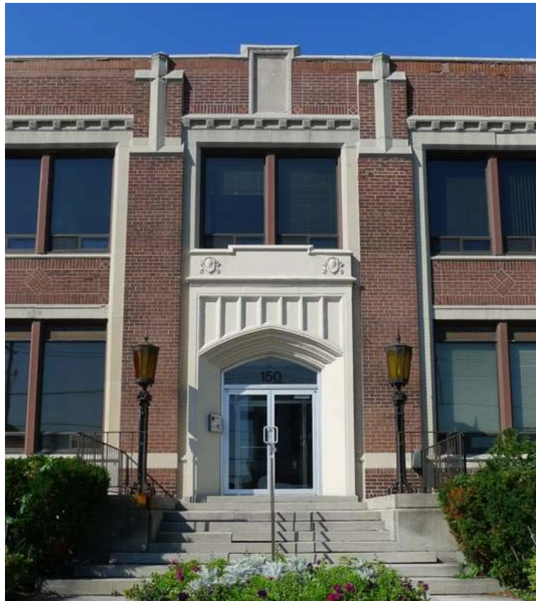
Showing the principal (east) façade of 150 Laird Drive (above) and principal entrance bay (below) ( Heritage Preservation Services, 2015 )
