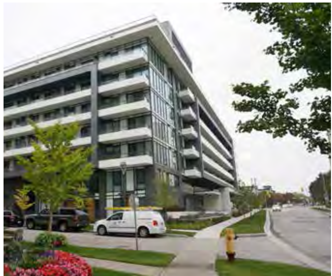
A network of varied streets and driveways to support a wide range of uses and activities
