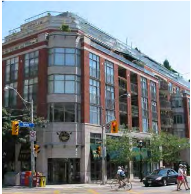
Mid-rise development with streetwall stepbacks and facade articulation to reduce the perception of building mass to the pedestrian
