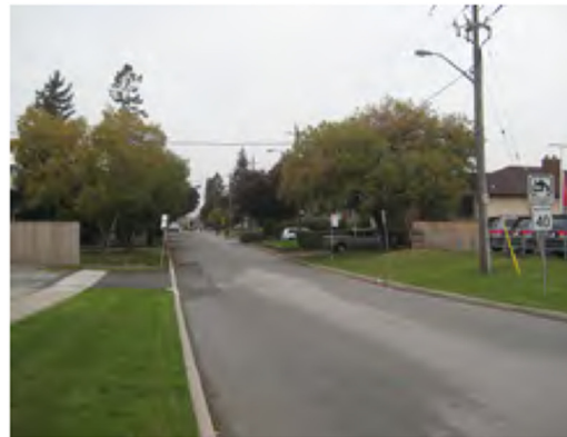
Some of the local streets have discontinuous or no sidewalks
