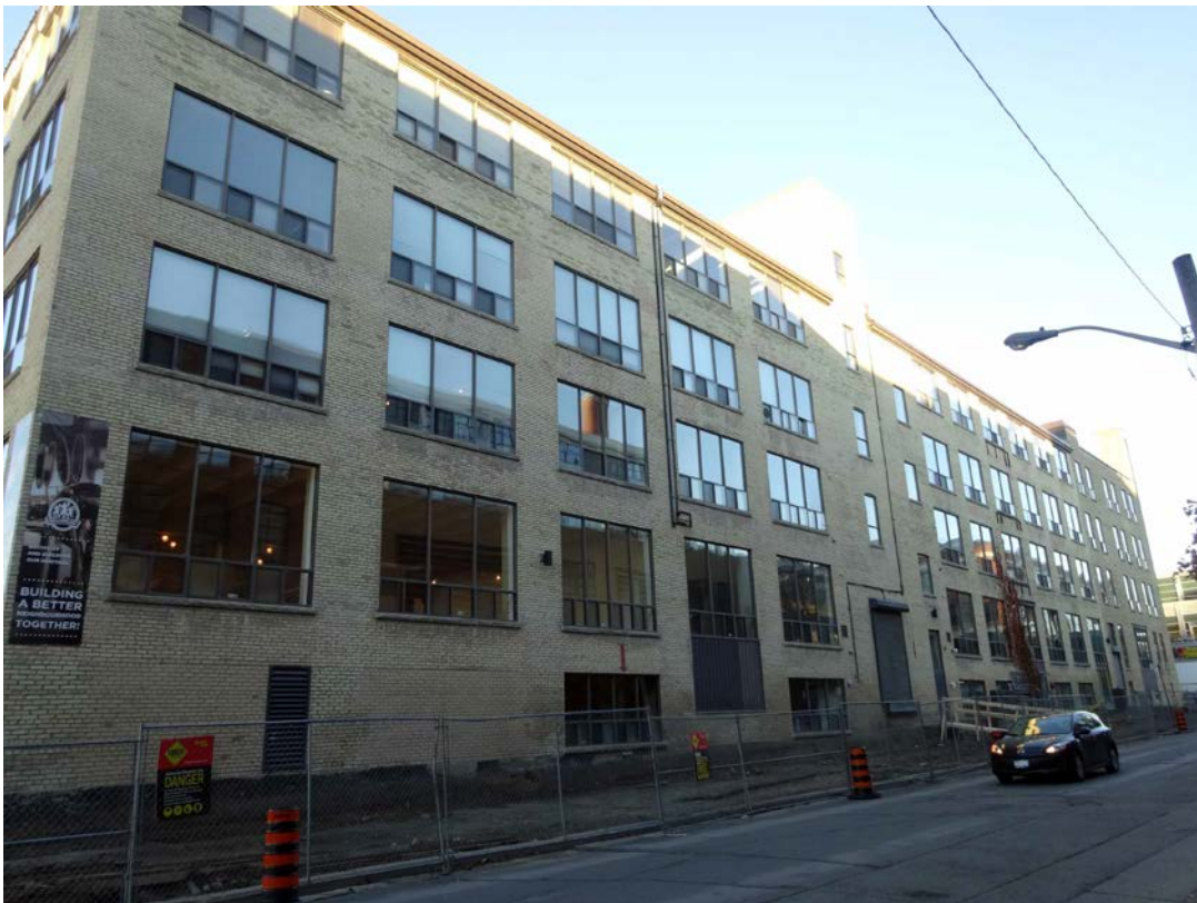
24. Current Photographs, 40 Hanna Avenue, 2014: in the top photograph the south (left) and east (right) elevations are shown, with the extended east elevation along Hanna Avenue below (Heritage Preservation Services)
