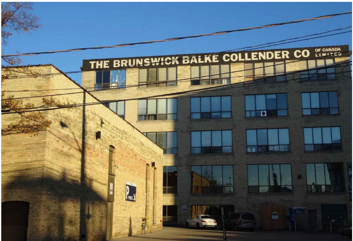
23. Current Photographs, 40 Hanna Avenue, 2014 : showing the west elevation of the 1912 section of the factory complex (above) and the south wall with the restored painted signage and its proximity to the neighbouring boiler house (below) (Heritage Preservation Services)
