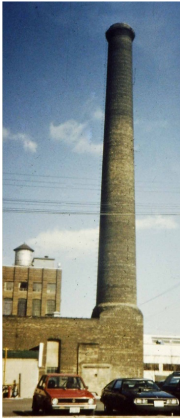
20. Archival Photographs, 40 Hanna Avenue, 1990s : showing the north elevation of the 1905 factory (above) and the west elevation of the boiler house with the landmark smokestack (below) (Toronto Historical Board)
