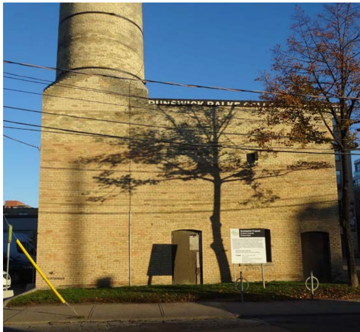
25. Current Photographs, 40 Hanna Avenue, 2014 : showing the boiler house from Hanna Avenue (above) and Liberty Street below) (Heritage Preservation Services)
