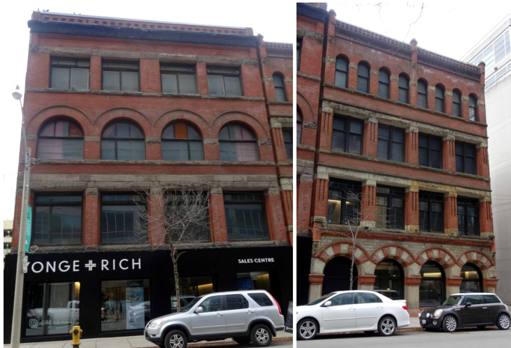
18. Current Photographs, 2014 : showing the south elevations of the properties at 26 Lombard Street (Heritage Preservation Services)
