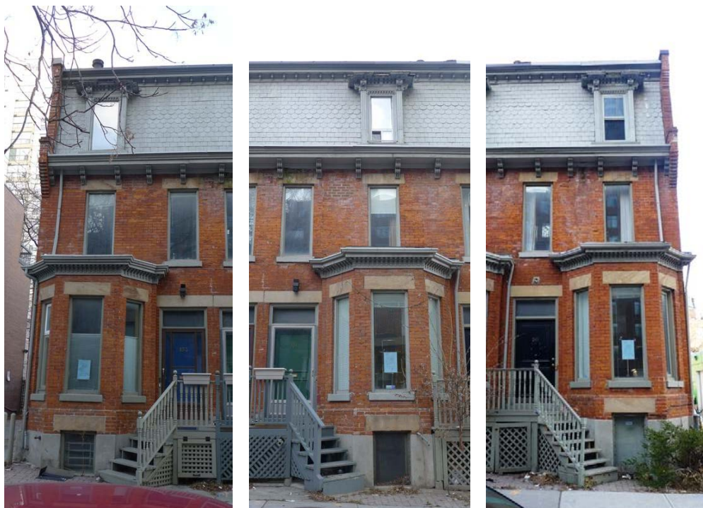
Showing the principal (west) façades of 193, 191 and 189 Mutual Street ( Heritage Preservation Services, 2014 )
