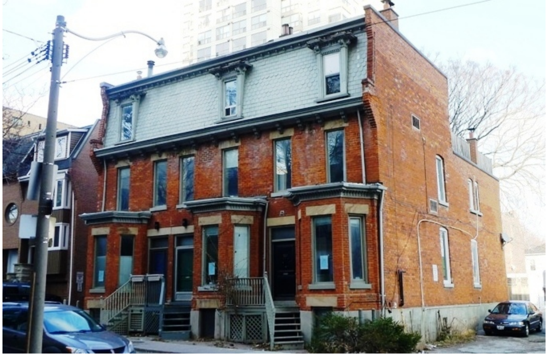
10. 193, 191 and 189 Mutual Street, 1887: showing the principal west and south elevations. ( Heritage Preservation Services, 2014 )
