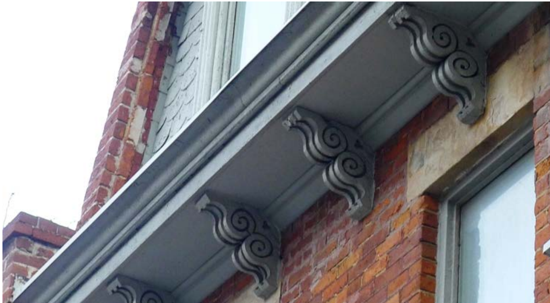
20. 193 Mutual Street : showing the cornice brackets with their incised scrolls supporting the soffit and eaves of the mansard roof. ( Heritage Preservation Services, 2014 )
