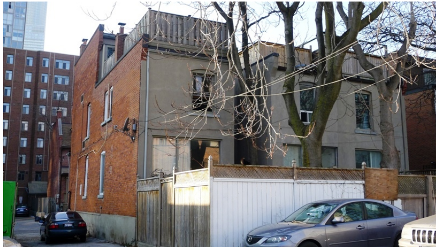
13. 193, 191 and 189 Mutual Street, 1887 : showing the south and west elevations with an indication of changes to the surface material and the windows at the first floor level. ( Heritage Preservation Services, 2014 )
