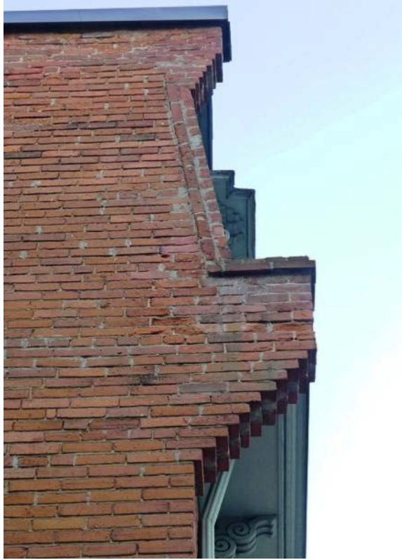
17. 193 Mutual Street : showing the corbelled firebreak wall at the second and mansard levels. ( Heritage Preservation Services, 2014 )
