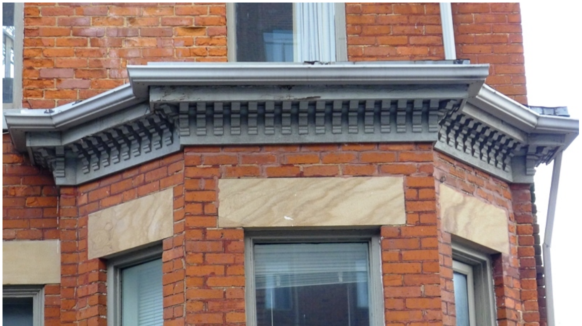
18. 189 Mutual Street, bay window detail : showing the limestone lintels and the richly decorated soffit of the eaves. ( Heritage Preservation Services, 2014 )
