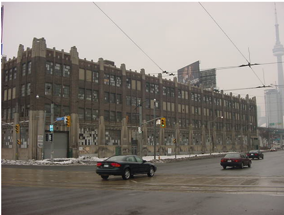
Loblaw Groceteria Building - South Elevation
