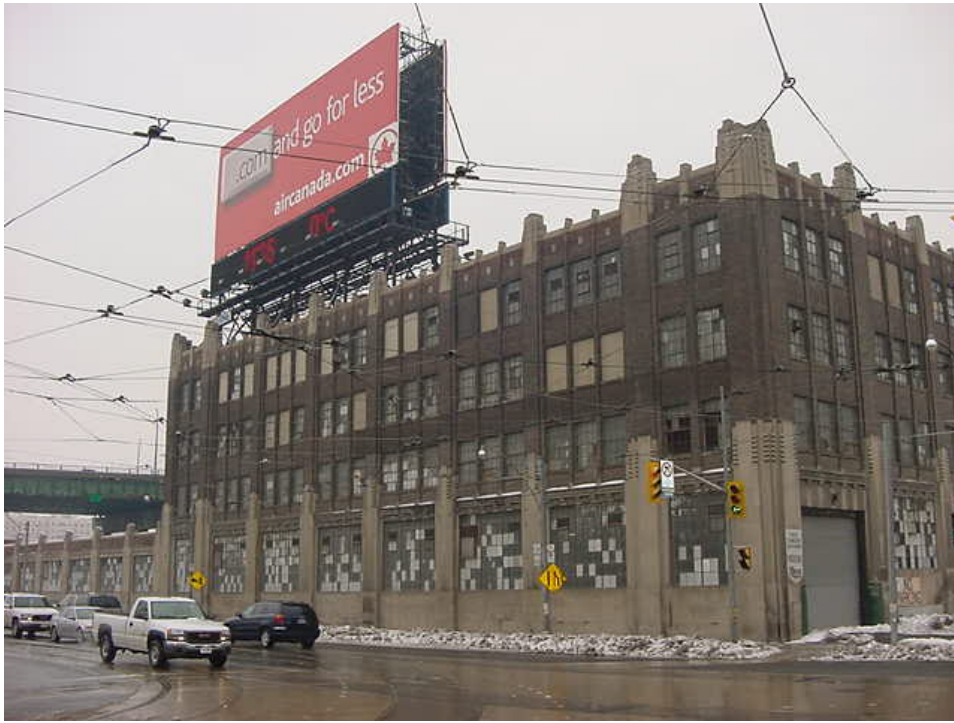
Loblaw Groceteria Building - West Elevation
