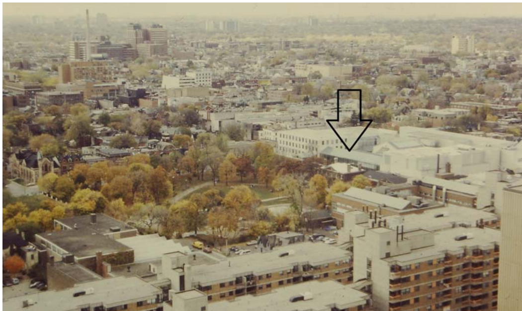
26. Aerial Photograph, 1994 : looking northwest and showing the Grange and Grange Park with the landscaped open space and, to the north the Stages I-III additions to the Art Gallery of Ontario (Toronto Historical Board)
