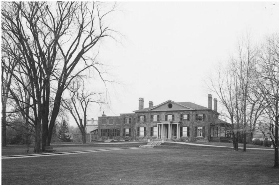
13. Archival Photograph, The Grange, 1897 : showing the Grange house raised with terraces, the verandah that replaced the conservatory at the east end (right), and the steps leading to the pathway to John Street across the grassed lawn (Toronto Public Library, Item 224)
