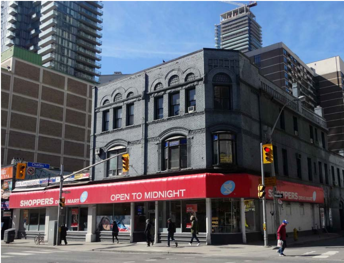
The Robert Barron Building (1889 and 1902) is the three-storey commercial building anchoring the southwest corner of Yonge Street and Charles Street West
