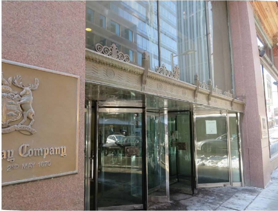
176 Yonge Street showing second bay of building on Richmond Street with non-original revolving doors, etched glass transom, and decorative bronze cornice.
