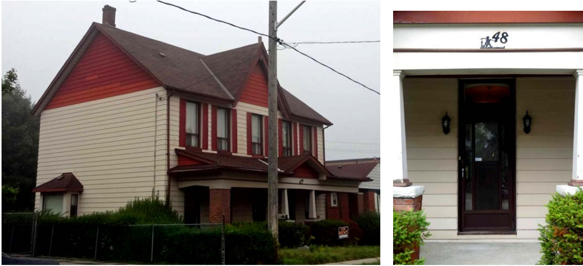
Above left: south wall with the bay window on the left; above right: main (east) entrance; Cover: principal (east) elevation of the Vivian House (Heritage Preservation Services, 2015)
