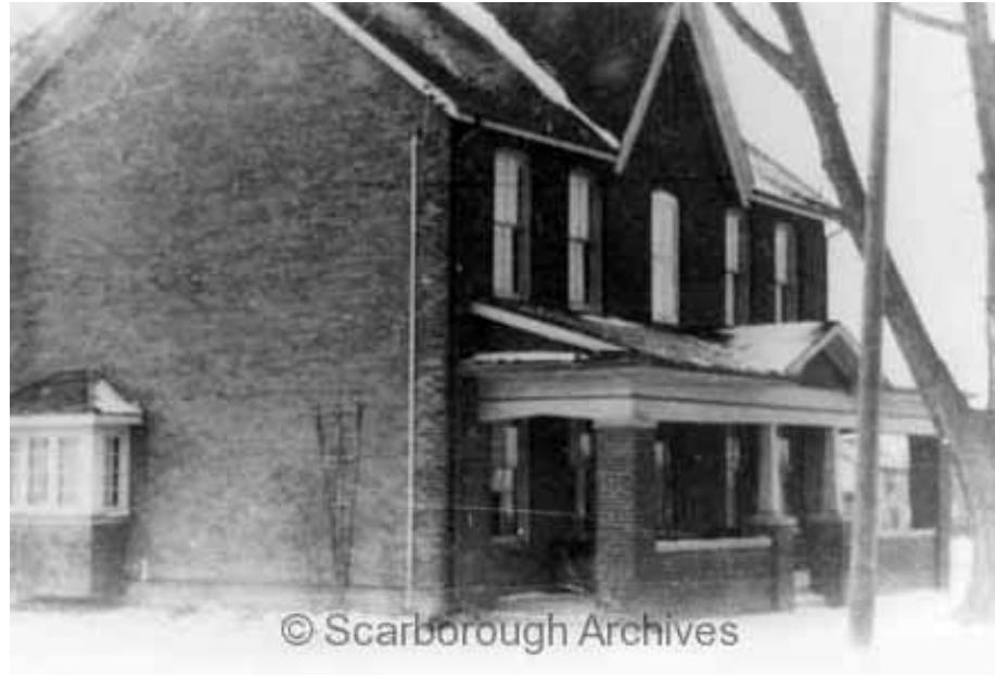
7. Archival Photograph, 48 Laurel Avenue, undated : showing the Vivian House with its brick cladding visible and following the addition of the bay window (left), which is not present in Image 6 above (Scarborough Archives as reproduced on http://scarboroughhistorical.ca ).
