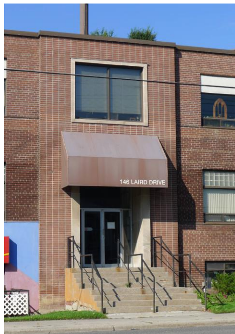
Showing the principal (east) façade of 146 Laird Drive (above) and principal entrance bay (below) (Heritage Preservation Services, 2015)
