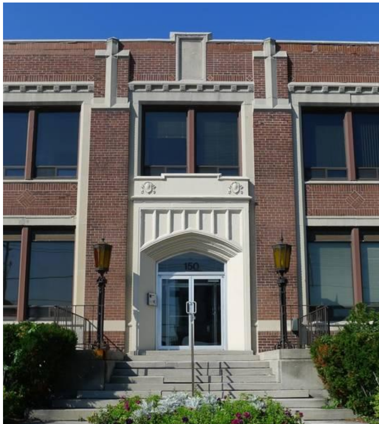
Showing the principal (east) façade of 150 Laird Drive (above) and principal entrance bay (below) ( Heritage Preservation Services, 2015 )
