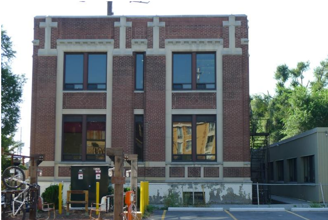
24. Durant Motors, north elevation : showing the narrow window bay between the two standard width bays. ( Heritage Preservation Services, 2015 )
