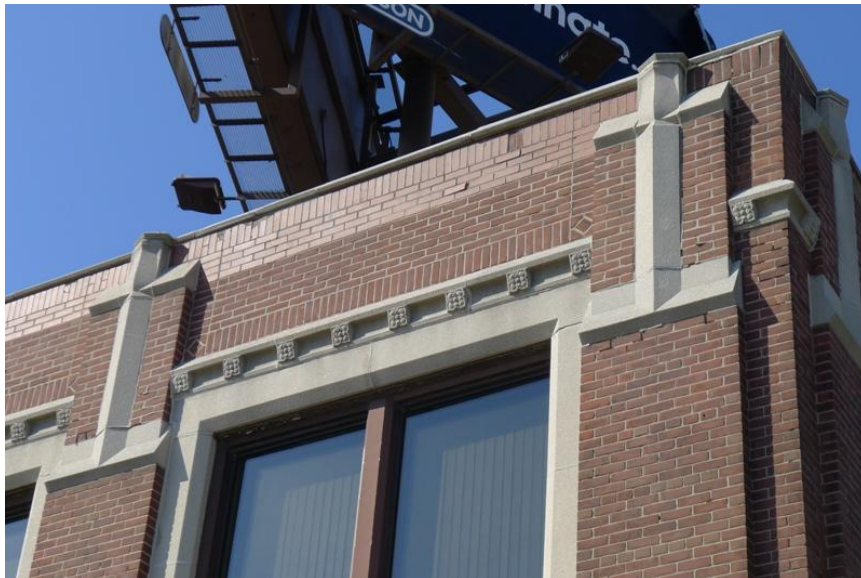
27. Durant Motors, east elevation detail : showing the cast-stone details of the buttress-like piers and the cast-stone surrounds of the windows with the decorative square bosses carved with rosettes and set below a protective drip mould as featured on the piers. ( Heritage Preservation Services, 2015 )
