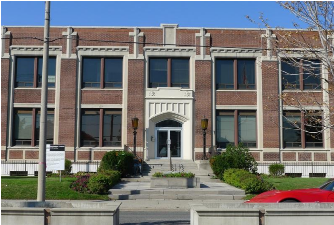
23. Durant Motors, east elevation detail. ( Heritage Preservation Services, 2015 )
