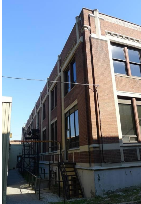
26. Durant Motors, west elevation : showing the same carefully detailed treatment for all elevations. ( Heritage Preservation Services, 2015 )
