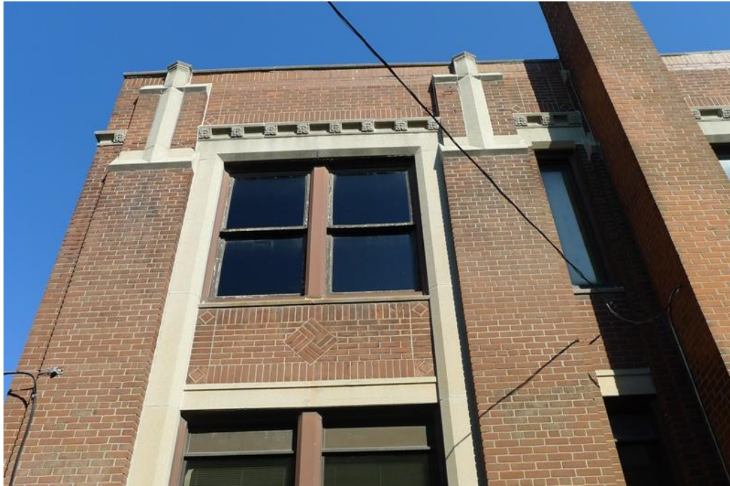
25. Durant Motors, south elevation detail : showing the chimney and narrow window as well as what appear to be original double-hung sash windows. (compare with Image 22) ( Heritage Preservation Services, 2015 )
