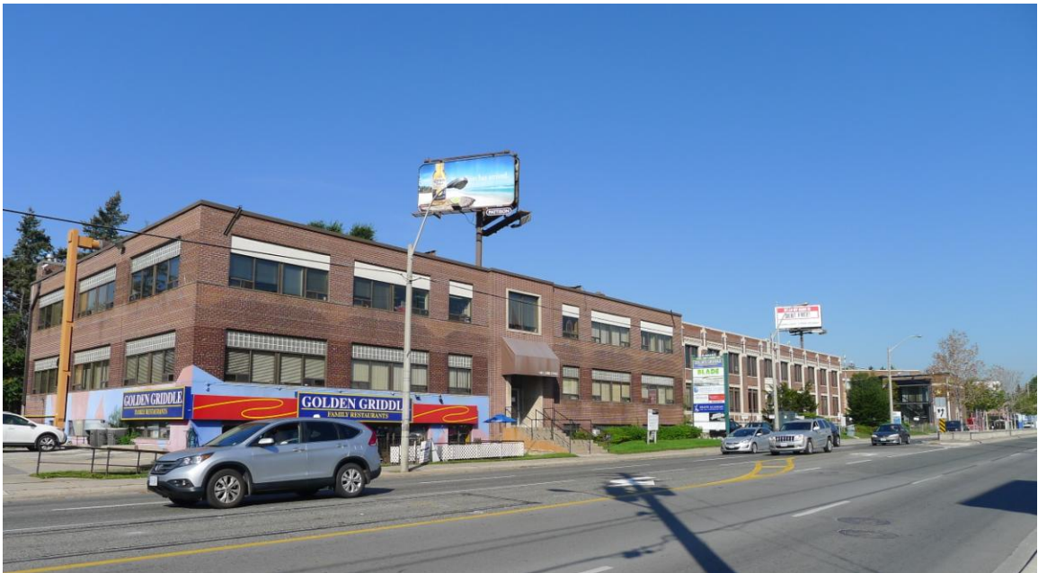
31. Laird Drive, east side looking north from Commercial Road : showing an office building at 146 Laird Drive (c 1959) initially rented to Imperial Oil and later occupied by the Metropolitan Separate School Board, Durant Motors at 150 Laird Drive and beyond, the former Imperial Bank of Canada at 180 Laird Drive. ( Heritage Preservation Services, 2015 )
