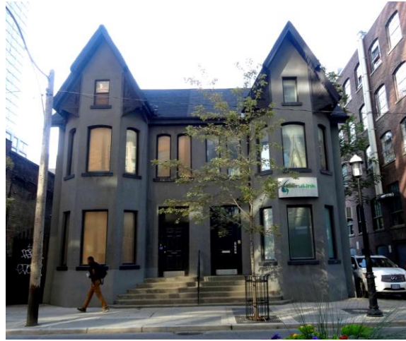
Principal (north) elevations, 357 and 359 Richmond Street West (Heritage Preservation Services, 2015)
