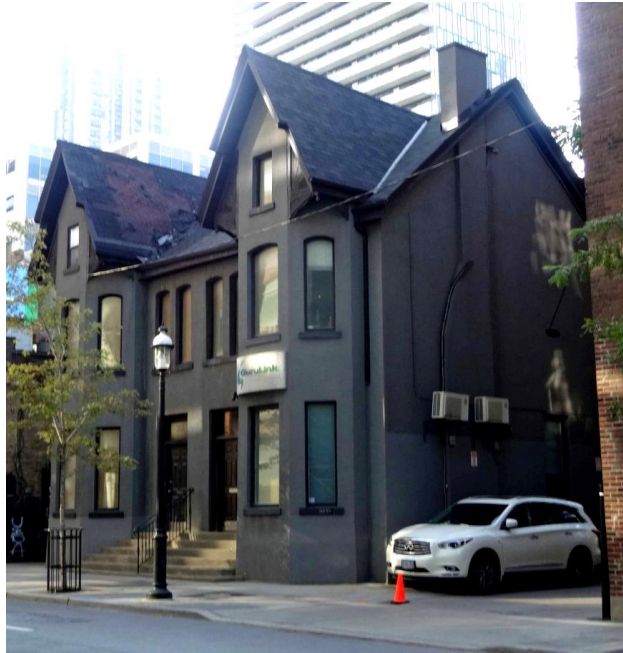
15. Current Photograph, 357 and 359 Richmond Street West, 2015 : showing the principal (north) elevations of the houses (left) and the west wall of 359 Richmond (right), which overlooks the laneway separating it from the adjoining 401 Richmond complex (Heritage Preservation Services).
