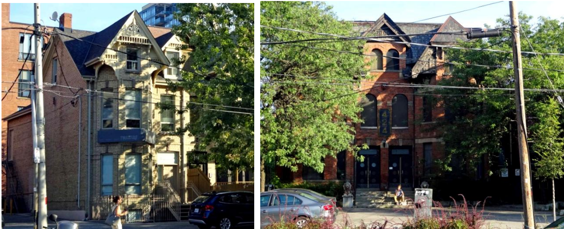
Above left: 374 and 376 Wellington Street West; above right: 422 and 424 Wellington Street West
