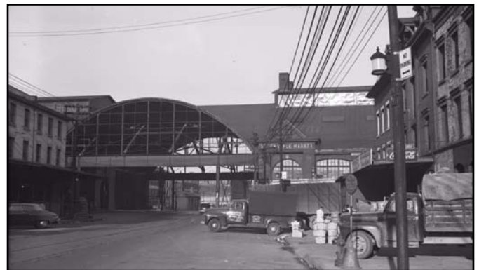
Figure 4: Demolition of the St. Lawrence Market's Front Street Canopy, 1952. Virtual Reference Library, Toronto Public Library.
