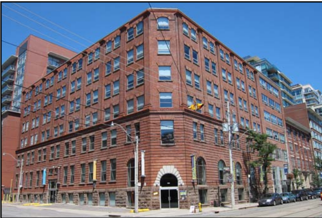
Figure 13: 204 King Street East, an example of a Industrial building
