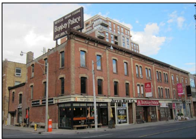
Figure 10: 61-75 Jarvis Street, examples of Commercial Warehouse buildings
