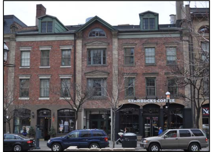
Figure 8: Polychrome brick, decorative stone detailing and ornamental storefronts at 81-83 Front Street East
