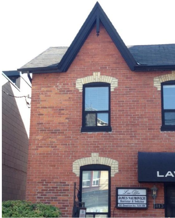
15. 813 Broadview Avenue: showing the decorative yellow brick window headers (Heritage Preservation Services, 2015)
