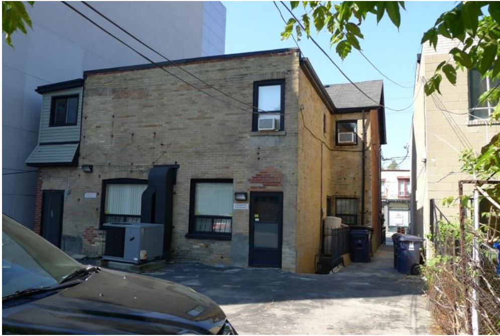
13. 811 and 813 Broadview Avenue, rear wing : showing the rear wing clad in yellow stock brick with a sloping flat roof. On the right, the side wall of the main house of 813 Broadview Avenue, clad in red brick with a gable roof. Note the later additions at ground and upper floors at 811 Broadview Avenue on the left ( Heritage Preservation Services, 2015 )
