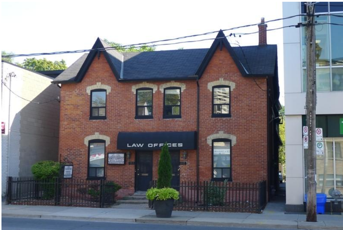
12. 811 and 813 Broadview Avenue, 1885-1890: showing the principal west elevation on Broadview Avenue ( Heritage Preservation Services, 2015 )
