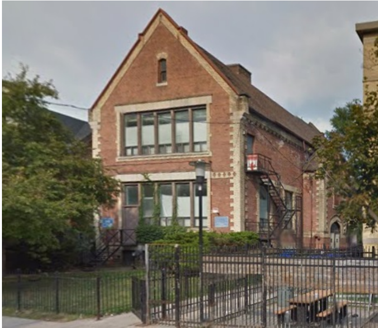
Current Photograph, 349 George Street
