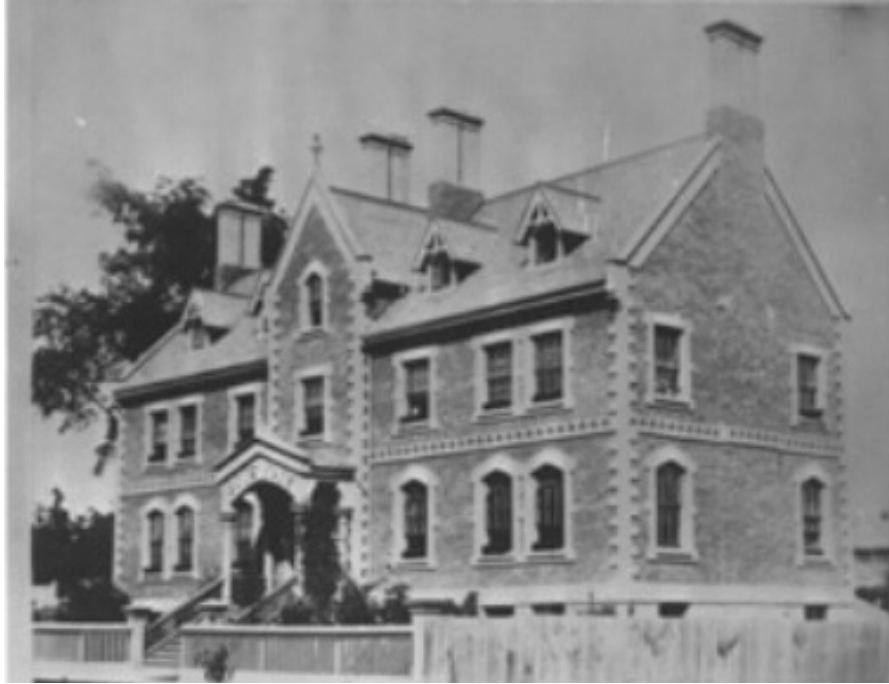
12. Archival Photograph, Toronto Boys Home, 1867 : showing the original building (1864) with the rectangular plan, gable roof with flared eaves, pattern brickwork, and central frontispiece containing the main entrance that are reflected in the design for the Allan School (Toronto Public Library, Item 11781).
