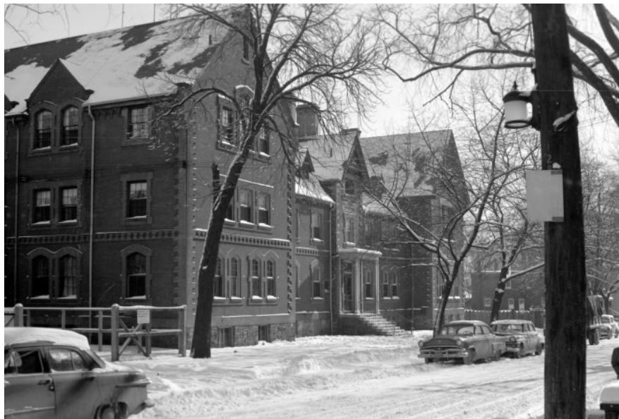
13. Archival Photograph, Boys' Home, 1954 : the institution is shown with its original building (centre), flanked by the late 19th century additions and prior to its replacement by Seaton House (Toronto Public Library, Item 764).
