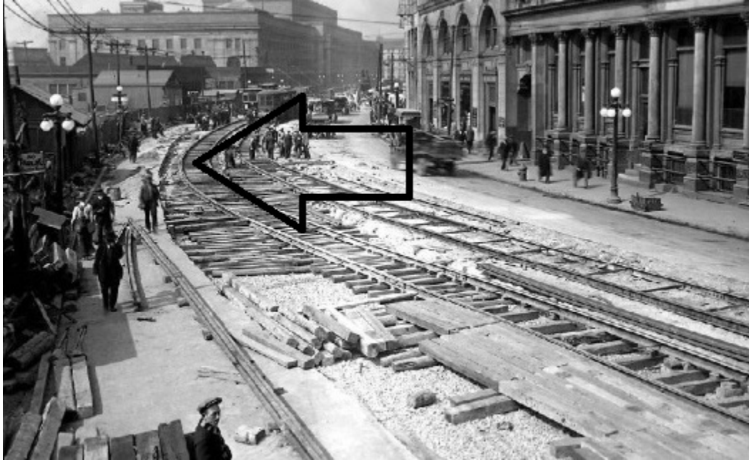
24. Archival Photograph, Dominion Public Building, 1930 : showing the excavation for the centre and east pavilions, with the recently-opened Union Station to the west (City of Toronto Archives, Series 71, Item 7597).
