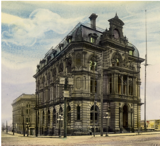
14. Archival Image, Customs House, 1910 : showing the 1873 building prior to its demolition (Toronto Public Library, Item 3949).
