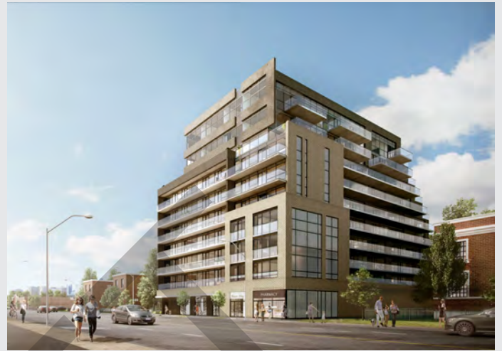
Facade along Danforth Avenue
