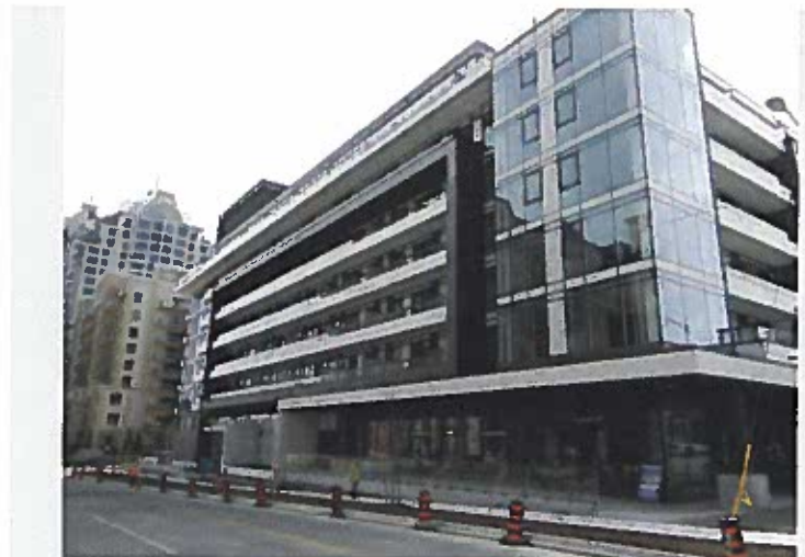
Facade along Rean Drive
