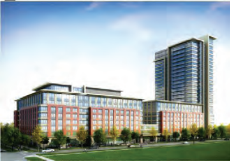
10 Under construction - a 24 storey senior's tower located 30m away from Steeles (does not have Steeles Ave East frontage) known as Mon Sheong with 6-8 storey base buildings.
