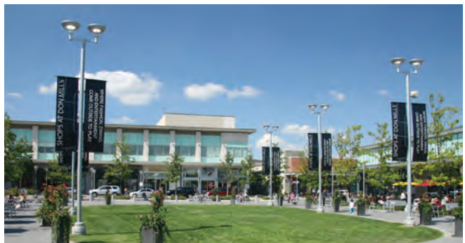
Shops at Don Mills: A retail-oriented open space features animated edges with public seating, and successfully works with retail frontages to create an active place.
