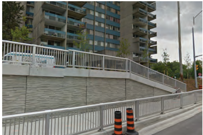
Sheppard Ave East and Kennedy Rd: Existing recently constructed underpass and retaining wall condition. For Steeles, a future grade separation would benefit from increased landscaped setbacks.
