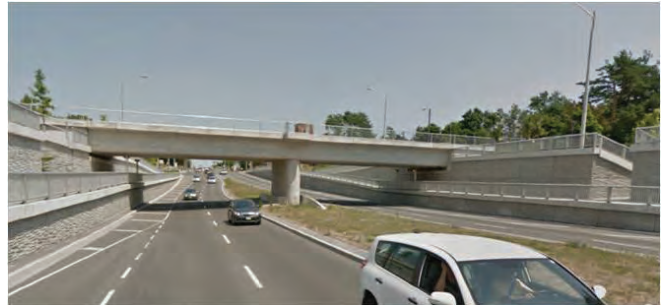
Sheppard Ave East and Kennedy Rd: Existing recently constructed bridge.
