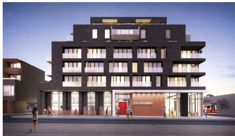
Facade along Manning Avenue
