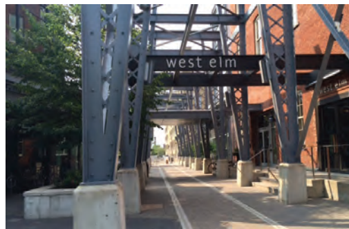
Mid-block walkway with adjacent retail and office uses - King St West near Hanna
