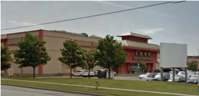
2 Splendid China and 4665 Steeles Ave Parking Lot
