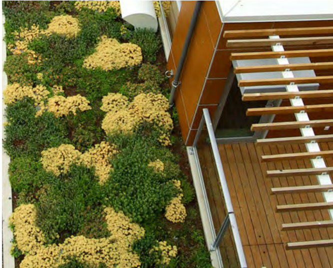
Green roof with native sedum mix. Credit: PWL Partnership Landscape Architects Inc.
