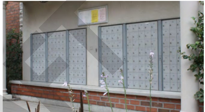
Good example of mail area integrated into building design with lighting and canopy.
