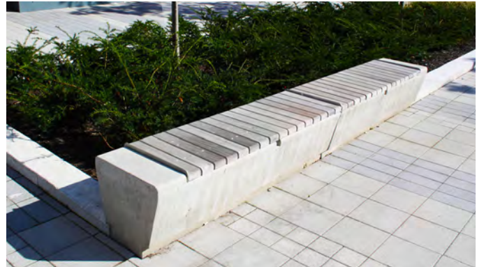
Well-designed seating bench integrated into landscaped planting bed.
