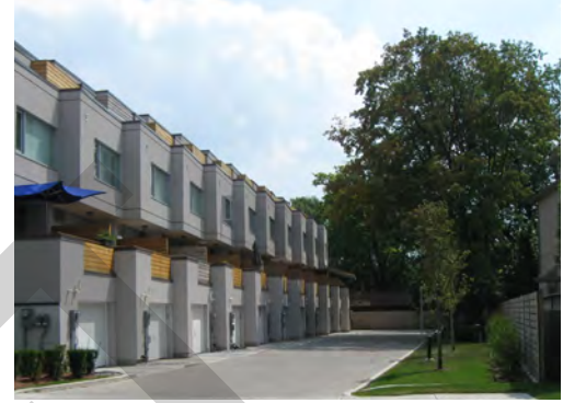
A generous landscape area along the rear property line provides buffer for adjacent property from new townhouses and garage and enhances the views from the townhouses
