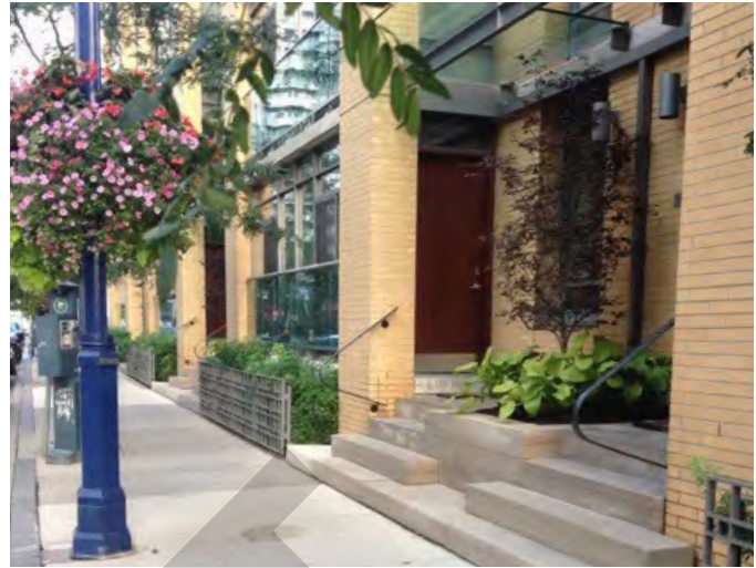
Well positioned and high quality doors, windows, and architectural details such as canopy, railing, screen, and planting areas all work together to enhance the public realm.
