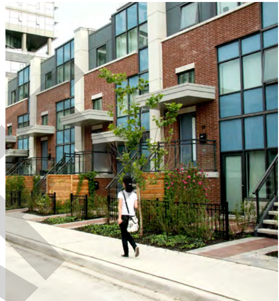
Accessible units are desirable in a stacked townhouse form. Internalize stairs to the upper units to reduce impact on streetscape and public realm.
