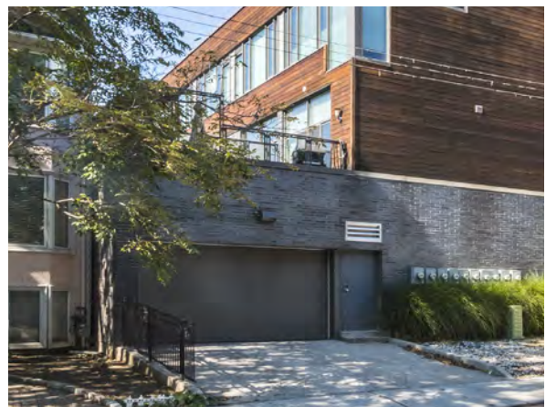
Internalizing parking garage into the building with private amenity space above is acceptable only if negative impacts such as shadow, privacy and overlook on adjacent properties can be limited and resolved.
