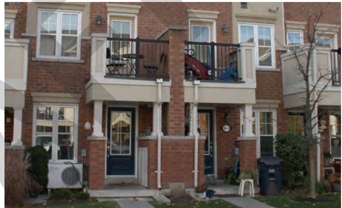
Example of building facade over cluttered with rainwater leaders, air conditioning units, utilities, and vents.
