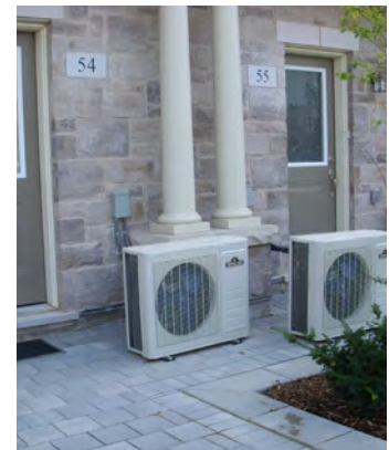
⊘ Poorly located utilities and mechanical systems adjacent to front entrance and street frontage negatively impact the quality and comfort of the public realm.
