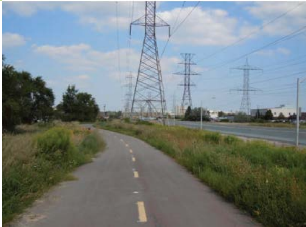
Figure 4: Sample Active Transportation Pathway / Multi-use Trail in Place of a Sidewalk on Roadway with Infrequent Crossings / Driveways. 177
