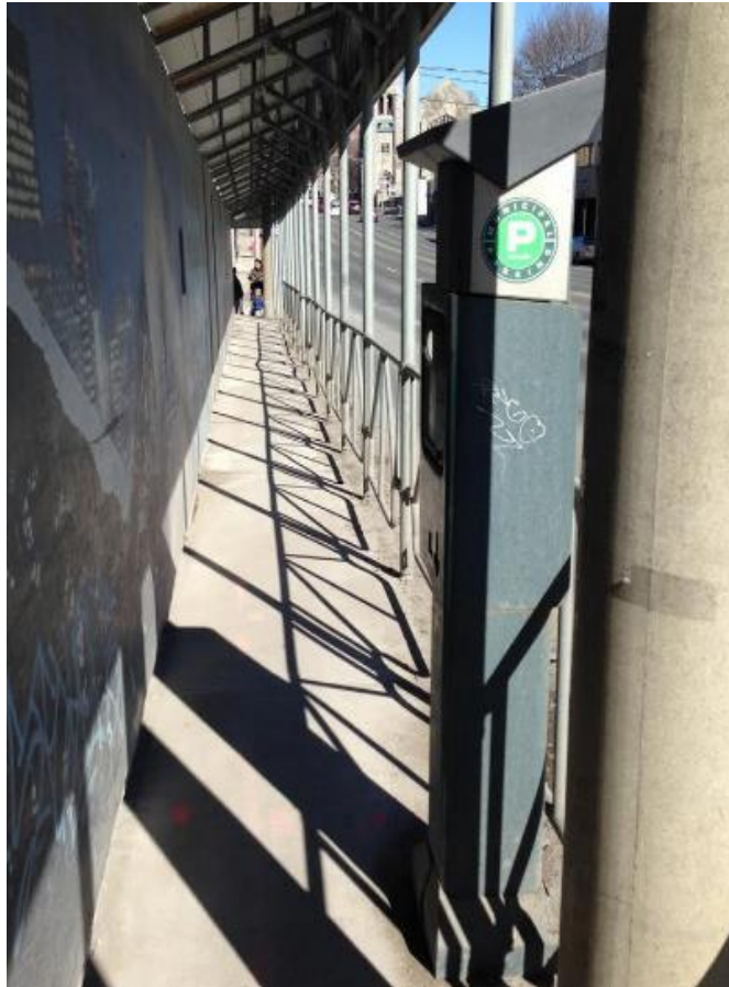
Figure 12 - ROW Occupancy with maintained TPA parking.
