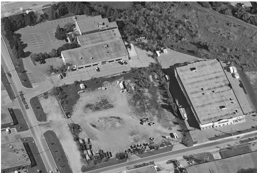
555 Ellesmere Road (upper left), 21 Principal Road (centre) and 100 Canadian Road (right)
