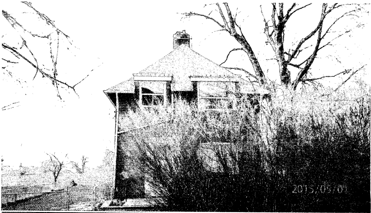
North Elevation of 17 Fishleigh Drive
