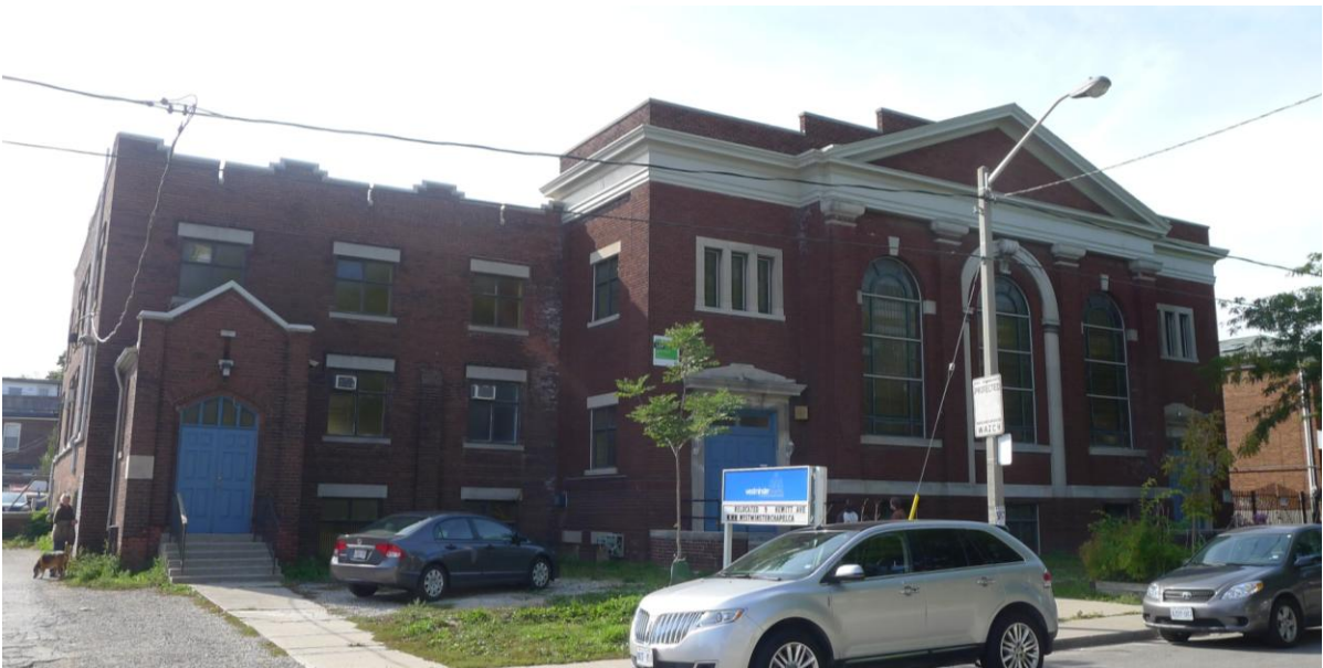
Showing the principal (east) façades of the 1913 (at the far left) and 1925 portions of the building complex on the west side of Dewhurst Boulevard (above, 1937, Temple Baptist Church and below, 2014, Heritage Preservation Services )
