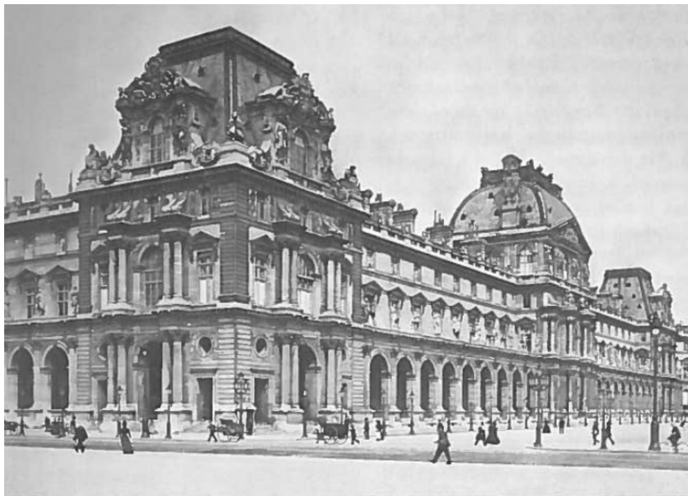
11. New Louvre, Paris, L T J Visconti and H M Lefuel, 1852-7: showing the mansard roofs and Classical Renaissance elements given the elaborate decorative treatment which typified the Second Empire Style. ( Hitchcock, p 195 )
