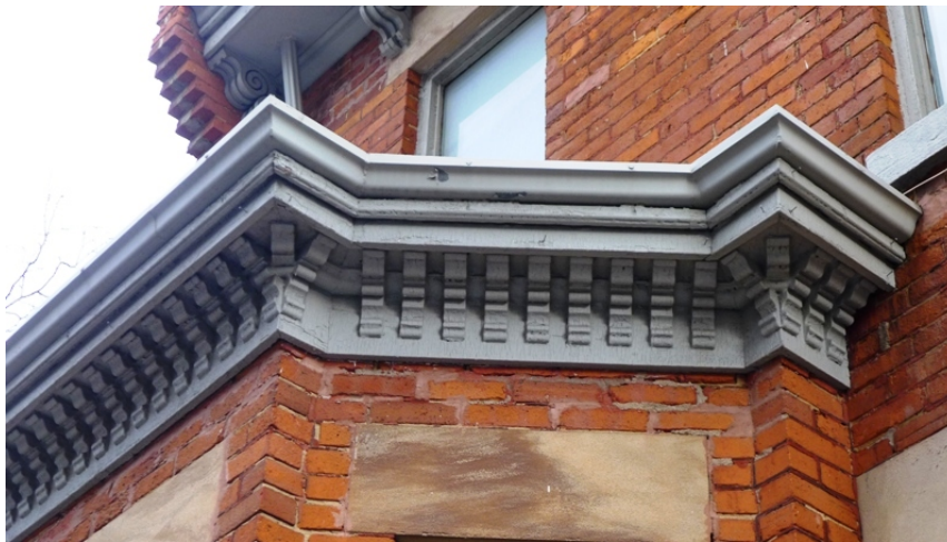
16. 193 Mutual Street : showing the precise construction of the bay window with the 90 degree-angle corners as transitions between the diagonal walls of the bay. ( Heritage Preservation Services, 2014 )
