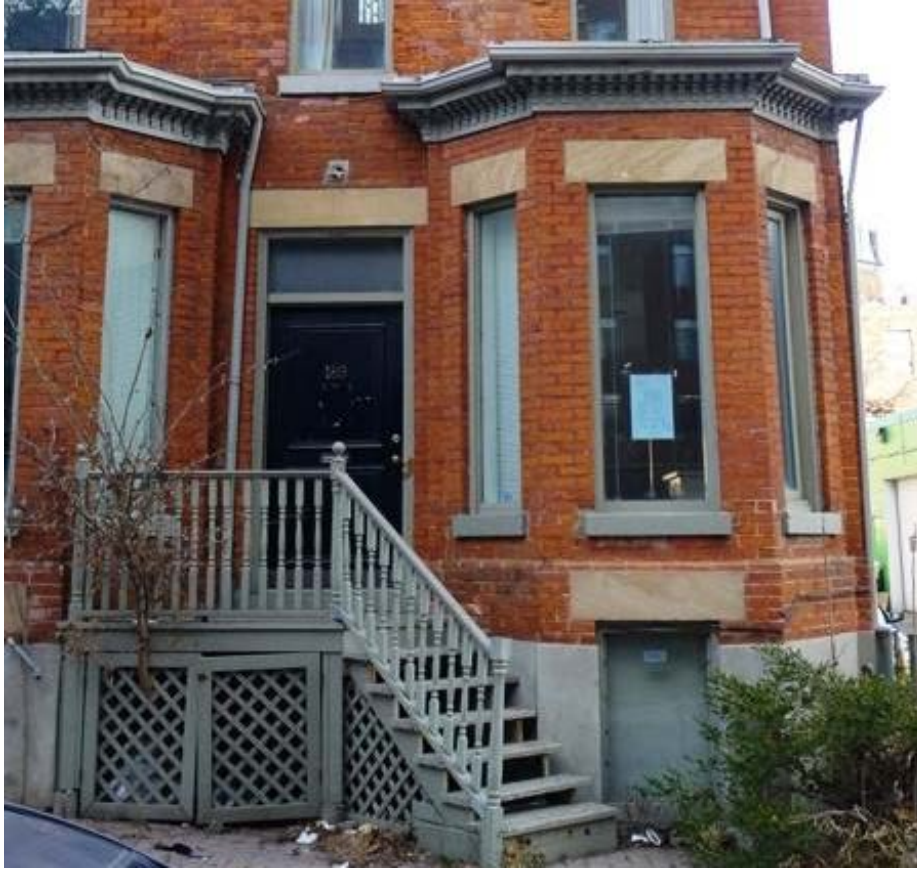
15. 189 Mutual Street : showing the projecting panel of brick above the raised stuccoed basement. ( Heritage Preservation Services, 2014 )
