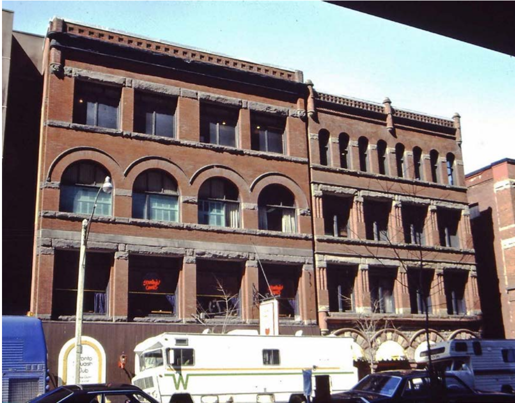
16. Archival Photographs, 26 Lombard Street, 1974 (above) and 1984 (below) : showing the placement of the subject properties on the north side of Lombard Street between Victoria and Church Streets (the former City Morgue and Lombard Street Fire Hall are visible in the distance, above), and the south elevations (below) (Toronto Historical Board)
