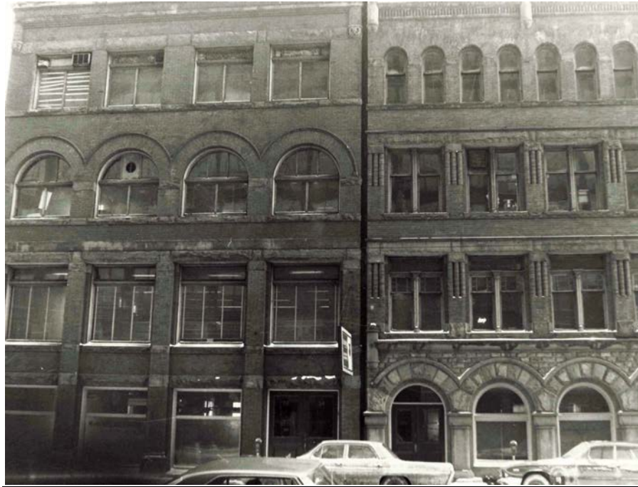
17. Archival Photograph, 1991 : showing the properties at 26 Lombard Street, including the first (ground) floor openings on the Barclay, Clark and Company Building (below left) that were subsequently altered (Toronto Historical Board)
