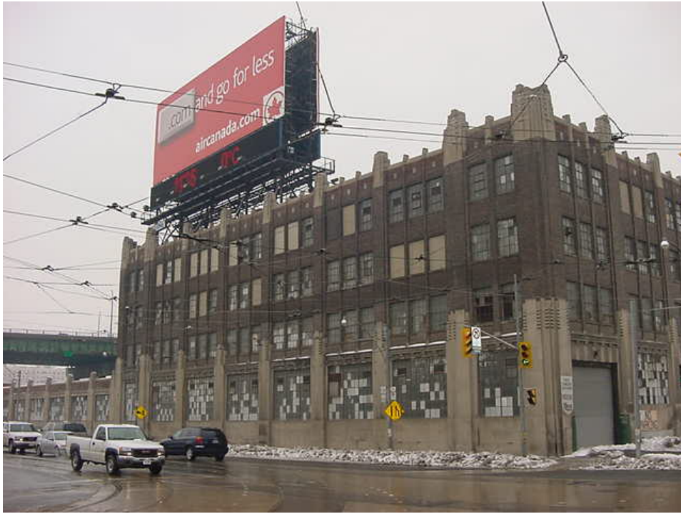
Loblaw Groceteria Building - West Elevation
