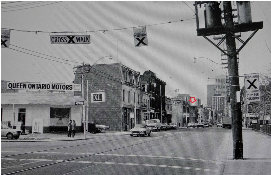
15. Archival Photographs, Queen Street East between Sherbourne and Ontario Streets, 1973 : showing the Andrew McFarren Building in its context on the south side of the street, east of Sherbourne Street (City of Toronto Archives, Fonds 2043, Series 1587, File 215)
