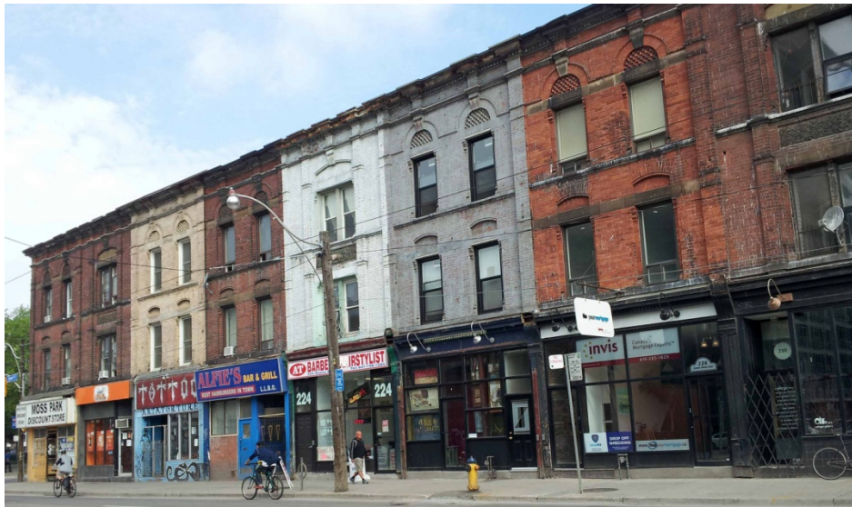
20. Contextual Photograph, 234-242 Queen Street East : showing part of series of commercial blocks (including the Carlyle Block, 1893) at the northeast corner of Queen and Sherbourne Streets, which were designated under Part IV, Section 29 of the Ontario Heritage Act in 1989 (Heritage Preservation Services, 2012)
