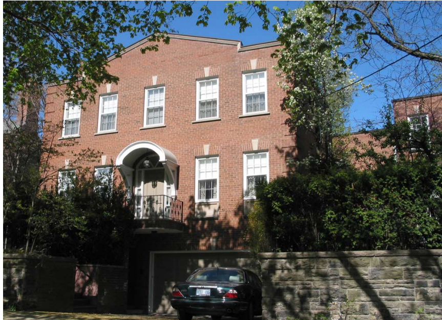
27 Cluny Drive- photo of existing 2-storey brick house
