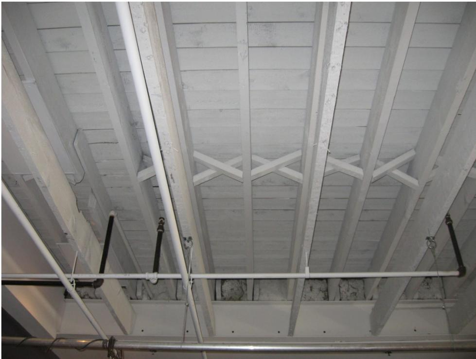
21. Stables interior roof structure: showing the combination of steel beams with wood structure. (*Heritage Preservation Services, January 2014*)
