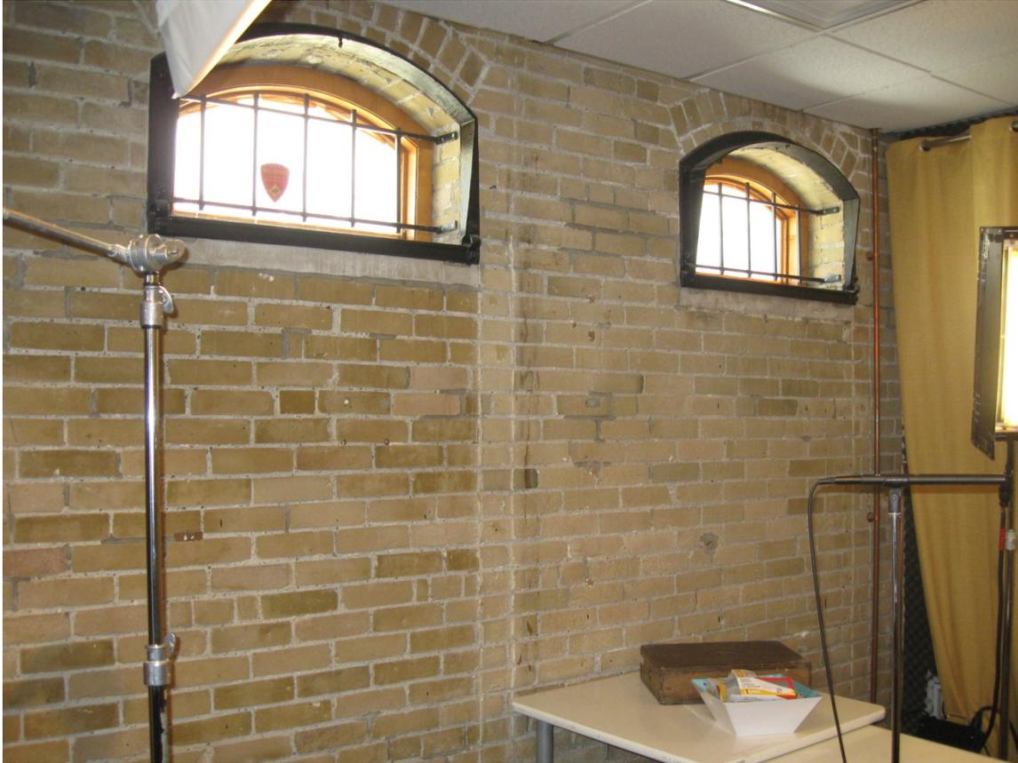
22. Stables interior: showing the original wall with evidence of stall partition and original metal framed windows with missing closing devices. (*Heritage Preservation Services, January 2014*)
