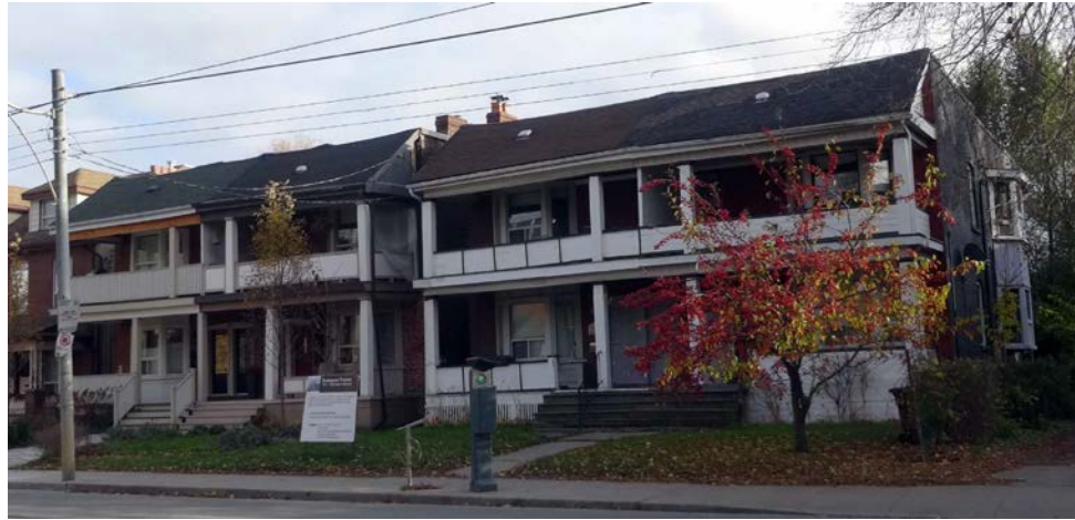
1333-1335 Queen Street East (right) and 1337-1339 Queen Street East (left) (Heritage Preservation Services, November 2014)
