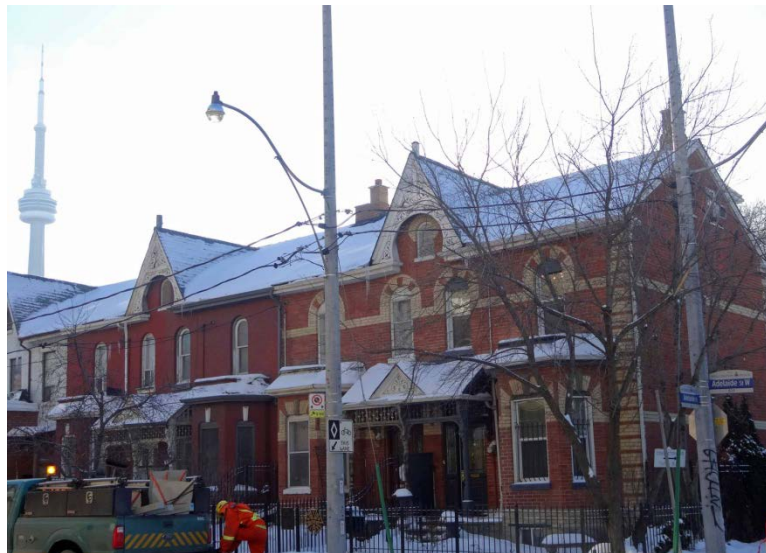
505-507 and 509-511 Adelaide Street West: William Clarke Houses
