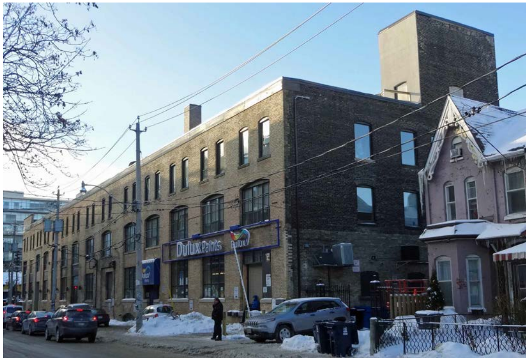
17. Current Photographs, 602 King Street West, 2015 : showing the south and west elevations (above) and the east and rear (north) walls (below) (Heritage Preservation Services)
