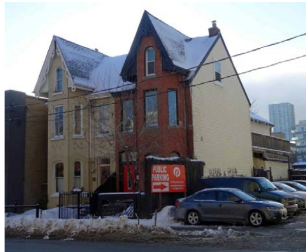
Above: view of the north (left) and west (right) elevations of the Marvyn Houses at 497 and 499 Adelaide Street West; cover: view of the principal (north) elevations of the houses (Heritage Preservation Services, 2015)
